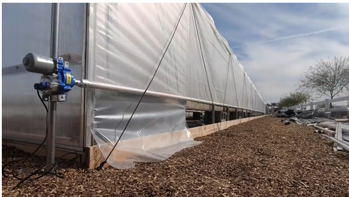
Image 44: Roller motor for a tunnel greenhouse that is equivalent to the greenhouses at Vegetable Garden de Haar 21
