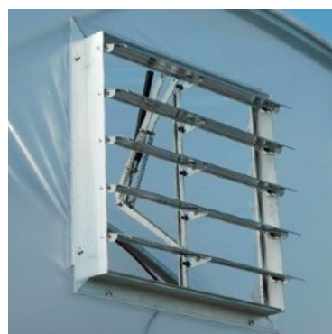
Image 41: Louvre window with automatic opening by means of cylinder
