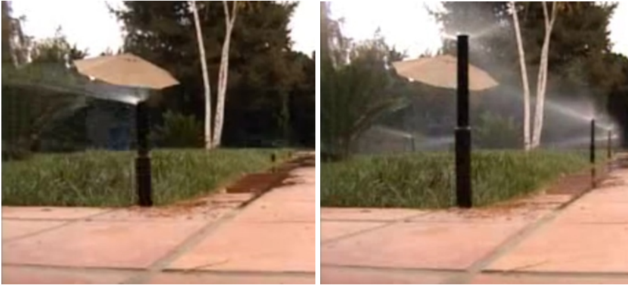
Image 70: These telescopic sprinklers rise when water pressure is applied 31,32
